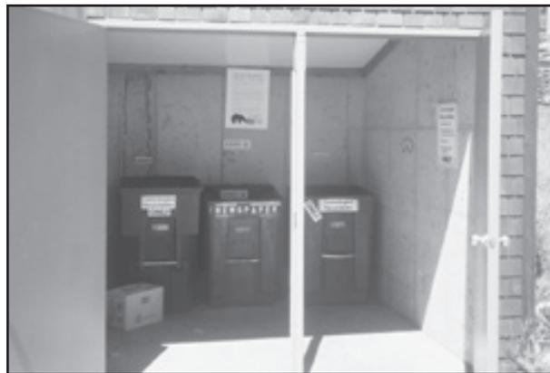
In areas with high bear activity, it's better to secure trash inside the house, in a sturdy locked garage, or specially constructed outbuilding with concrete or cinder block construction with heavy duty wood or steel doors and roof. Sides need to be flush with the ground, with no more than a 2-inch gap at the bottom of the doors. Ventilation holes should be kept to a minimum and covered with heavy-gauge steel mesh.
